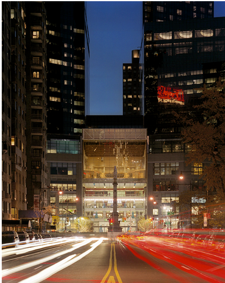
DOUBLE CABLE-NET WALL, TIME WARNER/JAZZ@LINCOLN CENTER, COLUMBUS CIRCLE, 59 TH STREET AND BROADWAY
